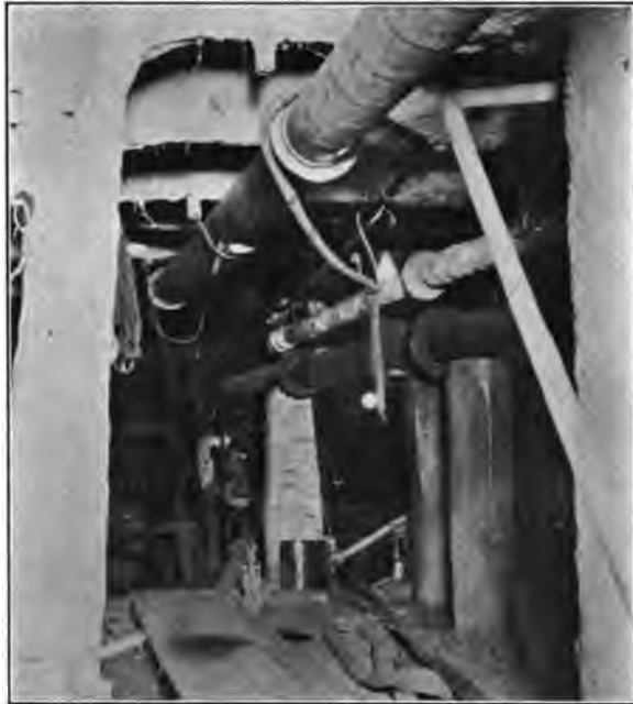
VIEW OF SUNDAY LAKE PUMP-HOUSE LOOKING TOWARD SHAFT
